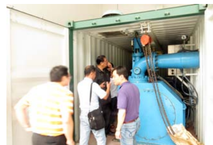
Visiting a containerized mini hydropower plant
